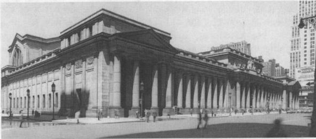
The Seventh Avenue façade of Penn Station looking uptown from West 31st Street. (Library of Congress)
